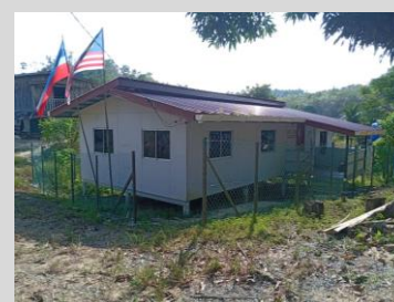
The school was able to build a new fence surrounding the building thanks to sponsorship support from SIRIM QAS.
