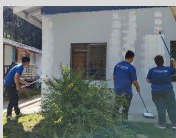
RedONE painting the school building during their visit to the school on 23 rd August.
