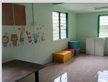
New floor tiling in the classrooms.
