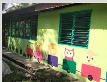
The outdoor walls had a fresh coat of paint and a beautiful mural.
